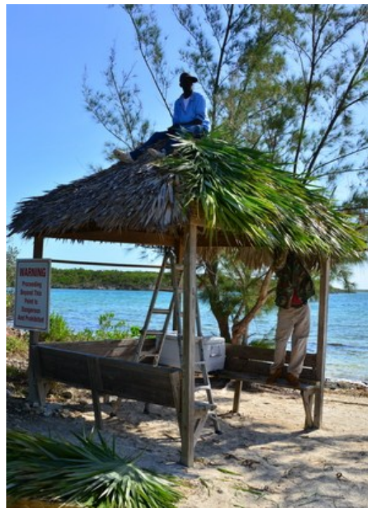
Re-roofing with green palm leaves
